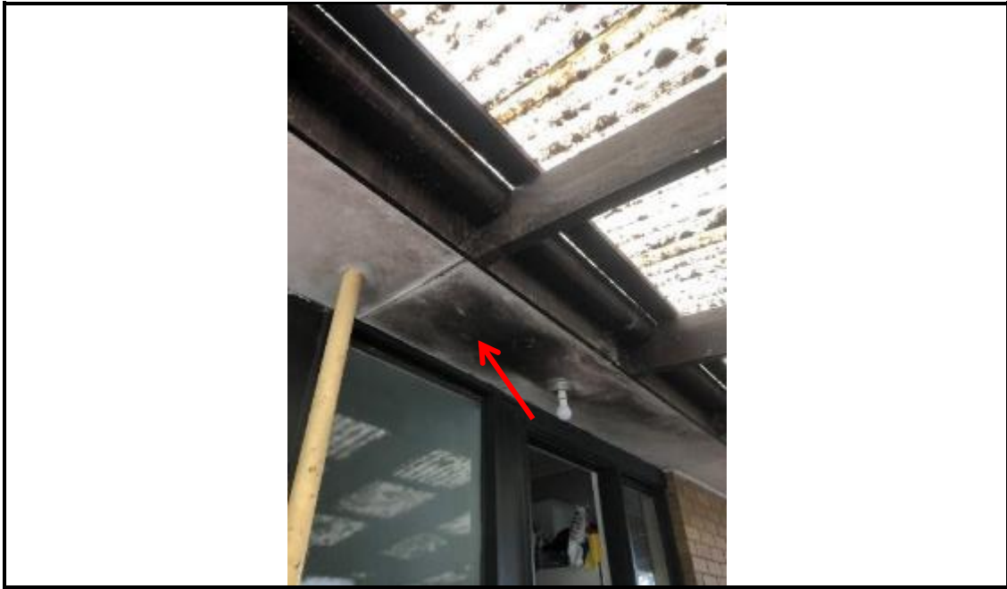
Photograph 5. Example of water damage to the eastern elevation ceiling lining.
