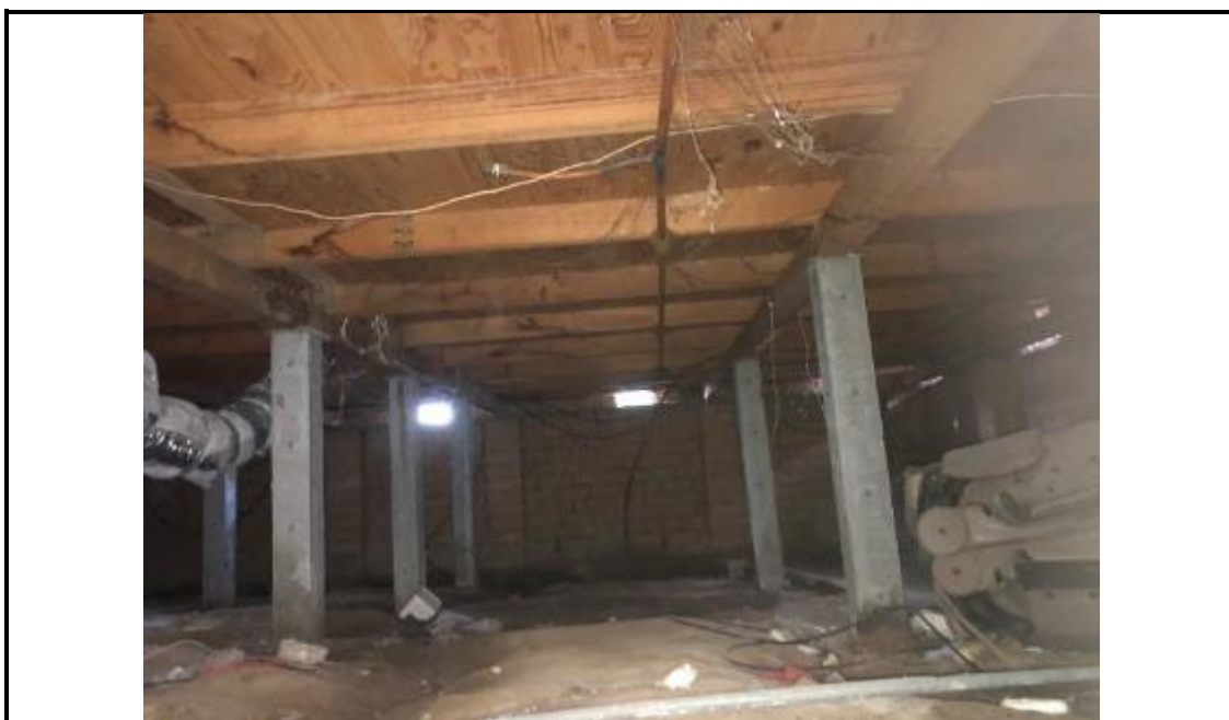
Photograph 7. Looking north from within sub-floor area.
