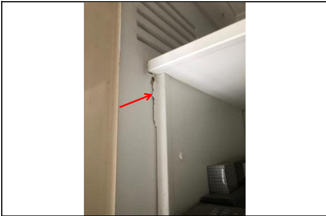
Photograph 15. Movement between master bedroom built in robe and adjacent wall.
