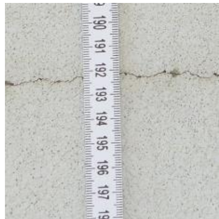
Photos 6 and 7 show the crack in the cold joint through the render.
