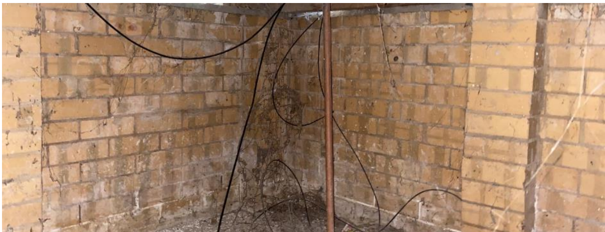
Photo 44 shows the north-western corner of the subfloor.
