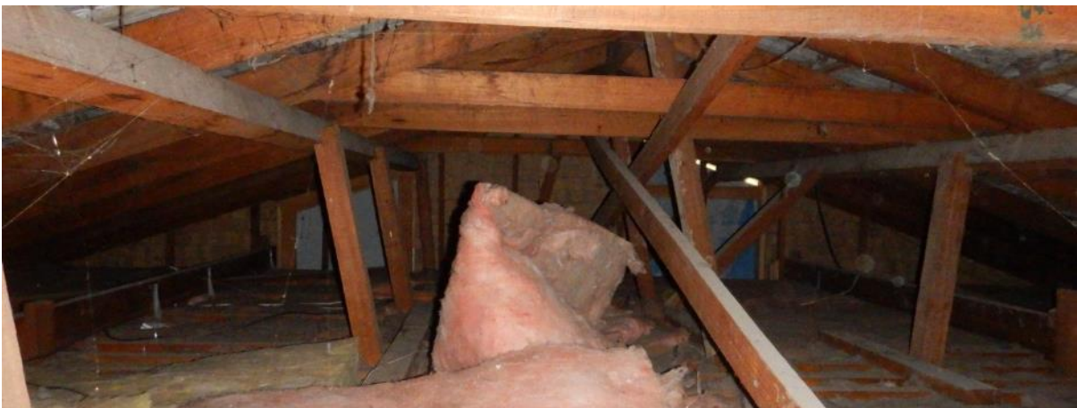
Photo 46 shows a typical view of the roof cavity.
