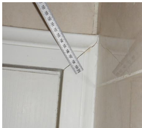
Photos 40 and 41 show the crack in the tiling and door architrave respectively.
