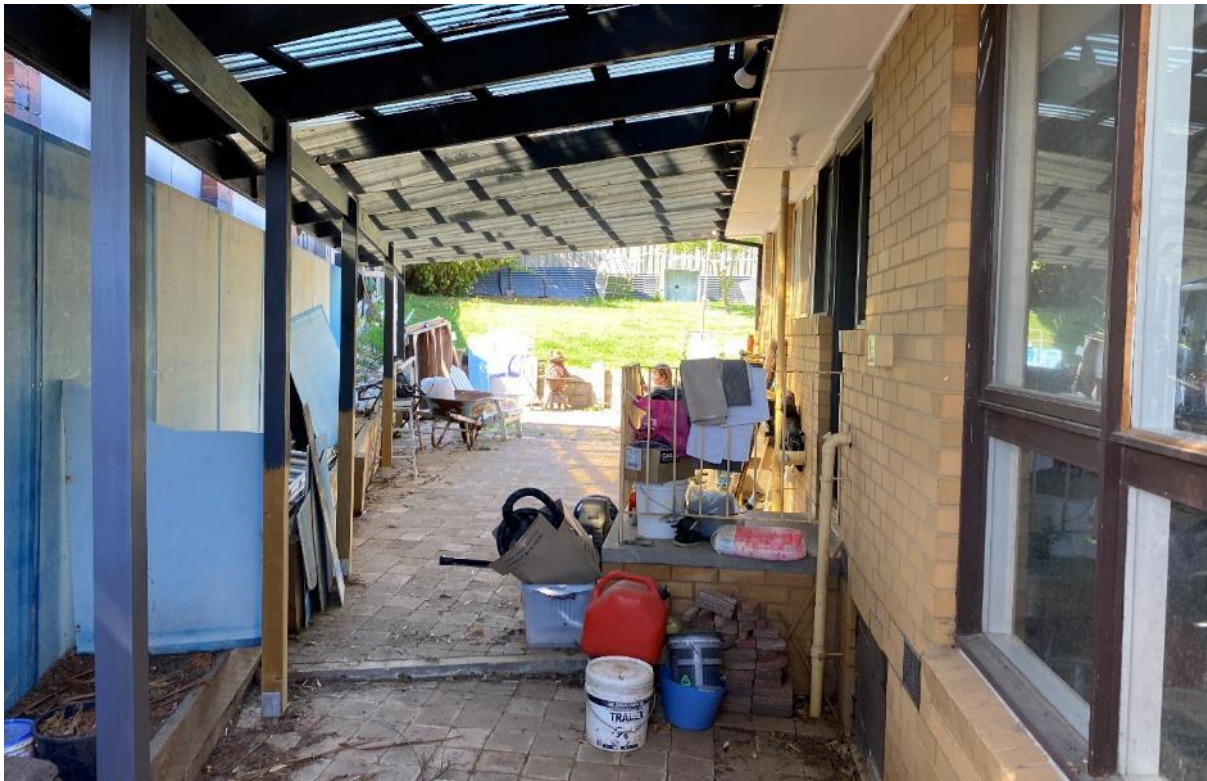
Photo 5 shows a typical view of the eastern elevation looking south.
