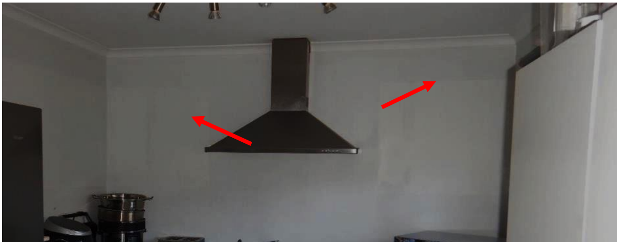
Photo 26 shows a typical view of the kitchen. Note the locations of the paint discontinuities where cabinetry was removed, and inadequate undercoat / primer was used.
