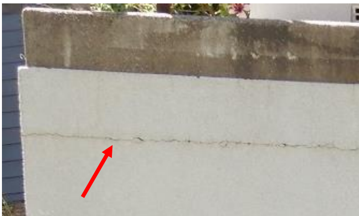
Photos 6 and 7 show the crack in the cold joint through the render.
