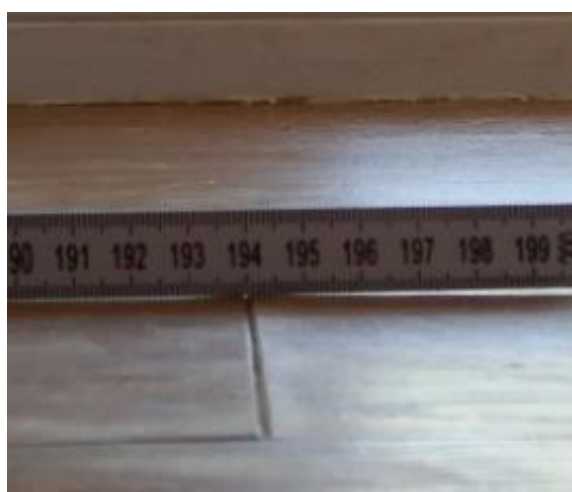
Photos 35 and 36 show examples of cupped floorboards.
