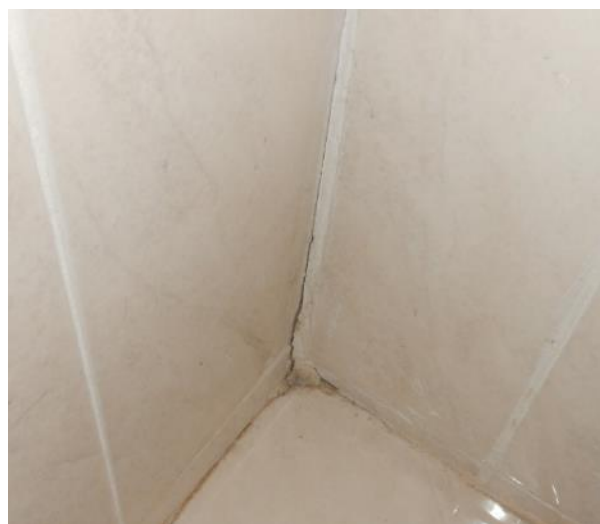
Photos 40 and 41 show the crack in the tiling and door architrave respectively.
