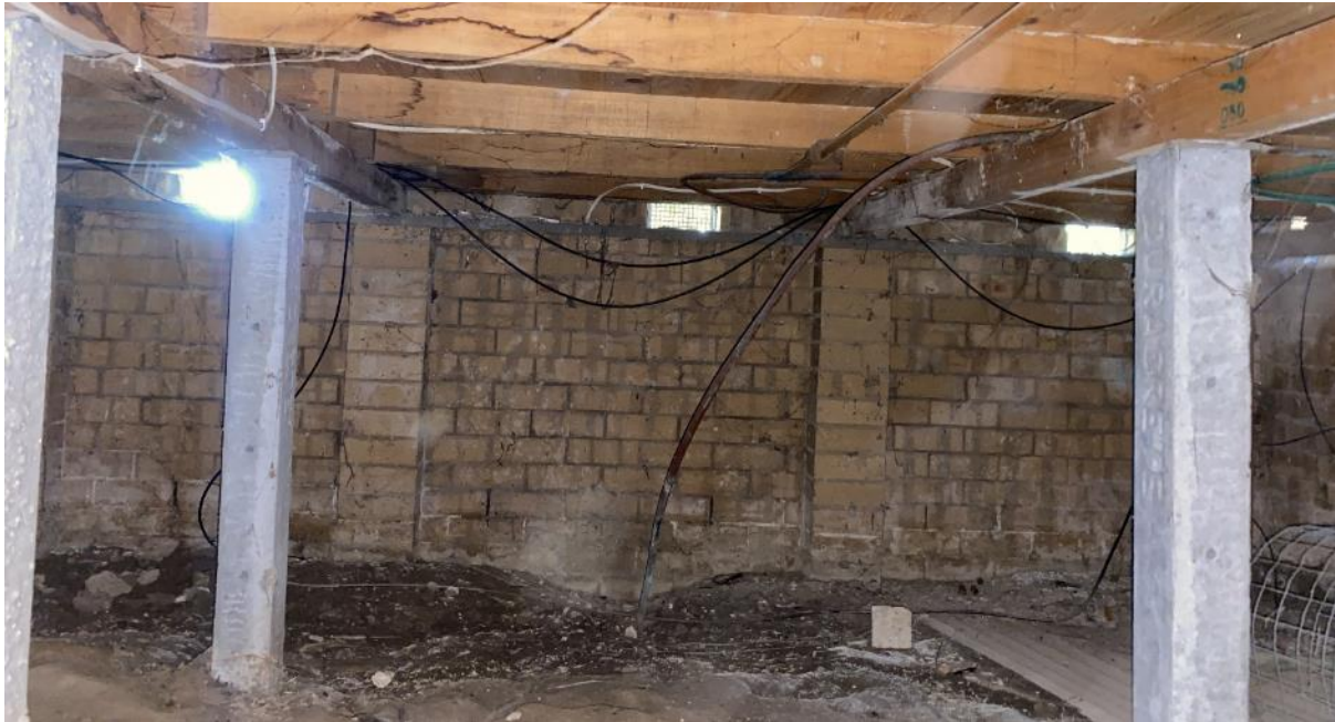
Photo 43 shows a typical view of the western sub wall.
