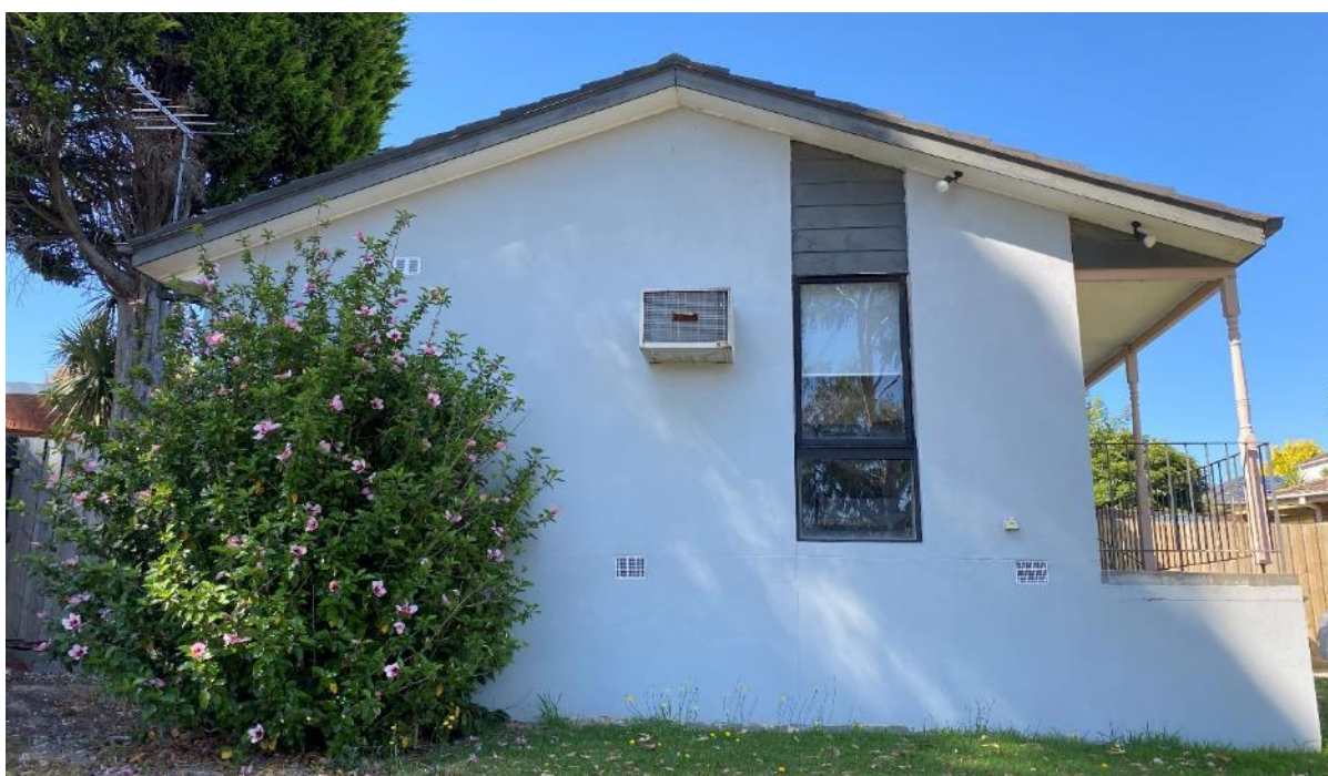
Photo 1 shows a typical view of the northern elevation.
