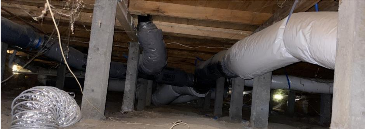
Photo 45 shows the centre of the subfloor cavity looking south.
