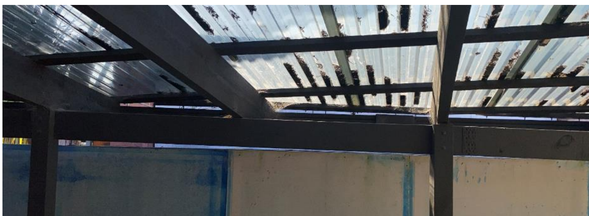
Photo 17 shows the underside of the timber pergola structure.
