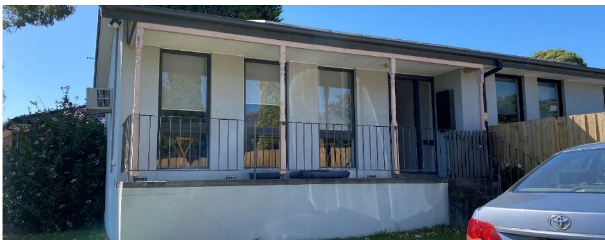
Photo 2 shows a typical view of the western elevation (northern end).
