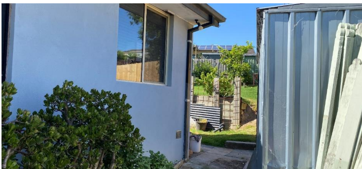
Photo 3 shows a typical view of the western elevation (southern end).
